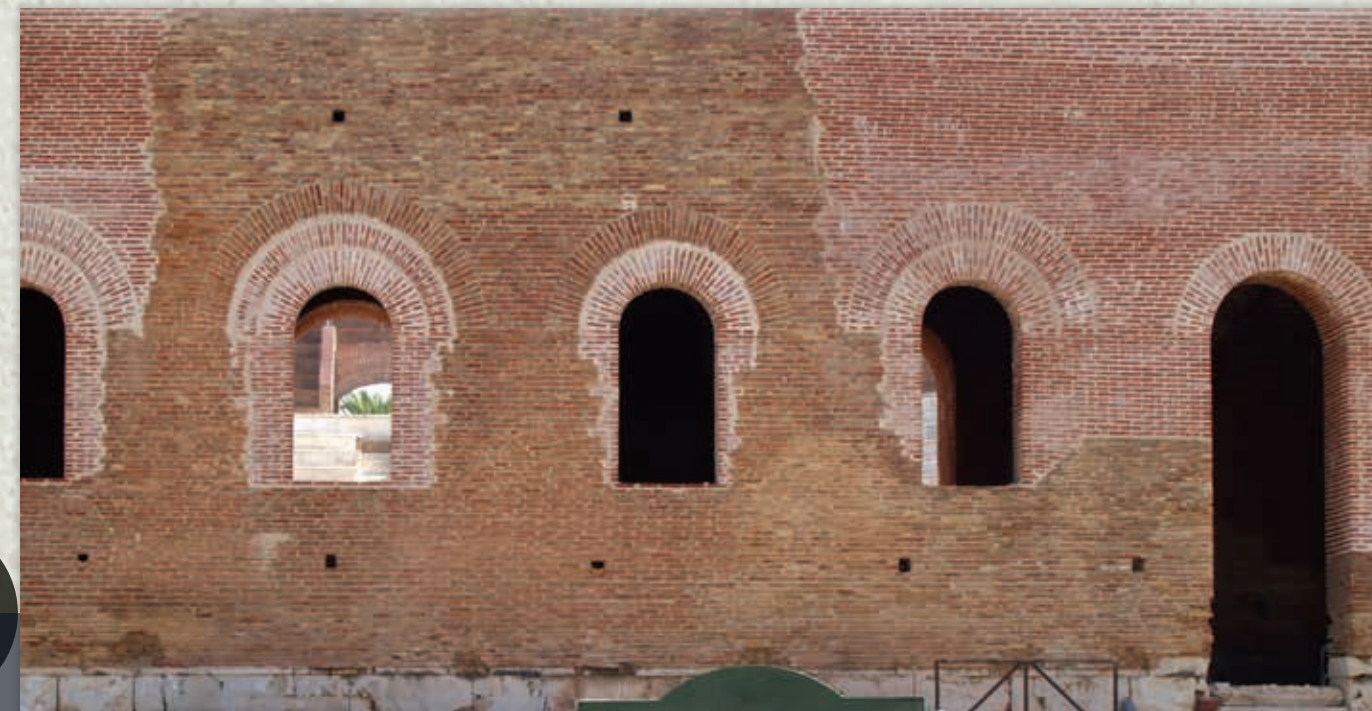
Windows on the south wall of the stage before and after the restoration
